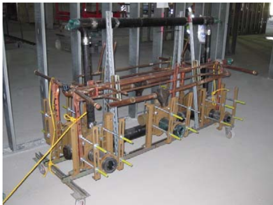
Water Closet Mobile Plumbing Carriers
