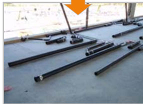
Prefabrication of waste lines
